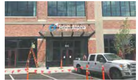
The new-construction office building is in the first phase of the Bottleworks project. (IBJ photo/Greg Andrews)
